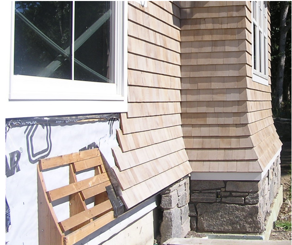
Picture of 4 piece 5.5" Radius flare with additional horizontal framing and fascia trim.
