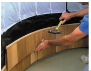
Overlapping End-Joints- patented panel construction design eliminates seams and prevents moisture penetration with no caulking between full panels.
